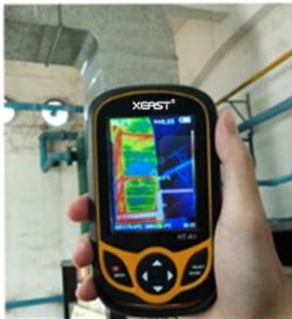
Check exhaust system
